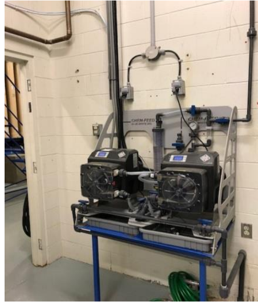
Images 7 and 8: Sodium hypochlorite generation system and pump skid
