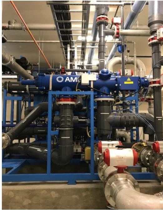
Image 2: Self-cleaning strainer
