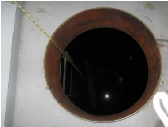
Images 9 and 10: Water Treatment Plant wet well access hatch
