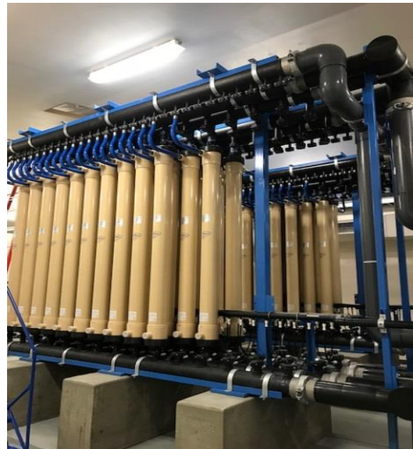
Images 3 and 4: Microfiltration modules
