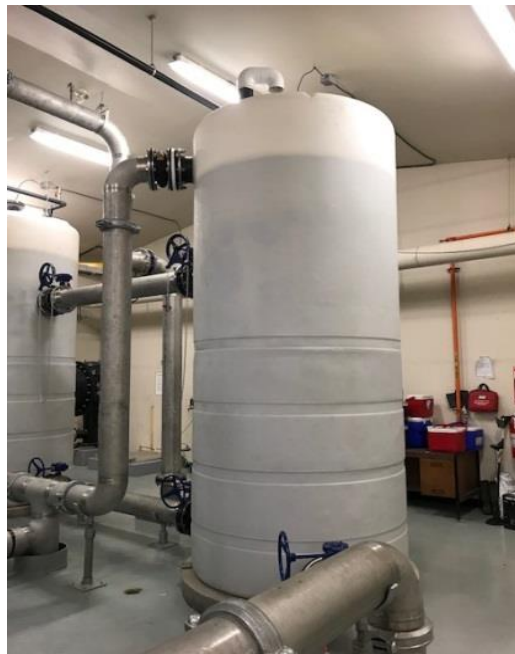
Image 1: Balancing tanks
