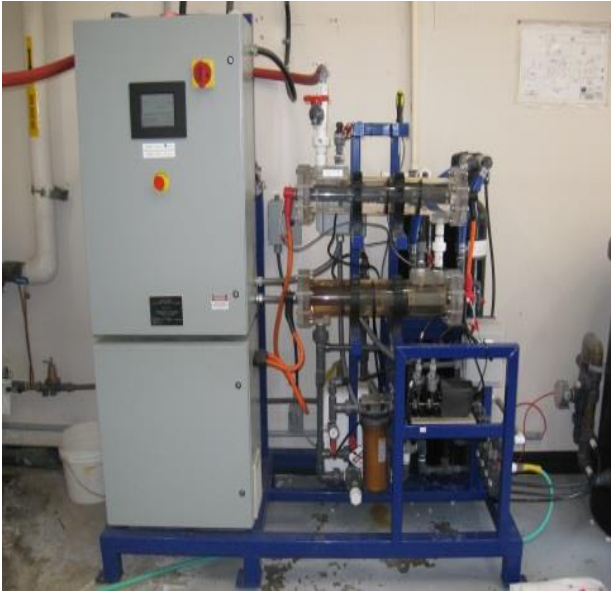
Images 7 and 8: Sodium hypochlorite generation system and pump skid
