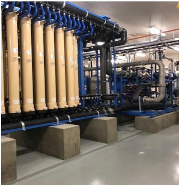
Images 3 and 4: Microfiltration modules
