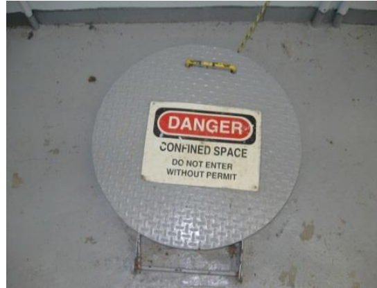
Images 9 and 10: Water Treatment Plant wet well access hatch
