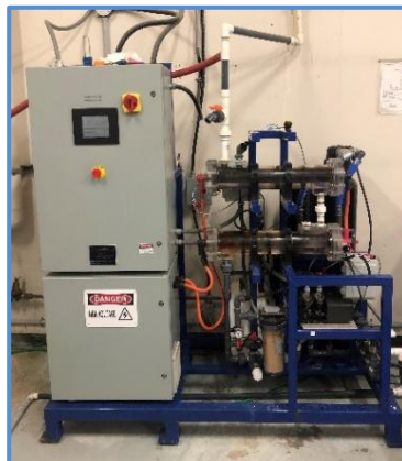
Figure 5. Sodium Hypochlorite Generation System
