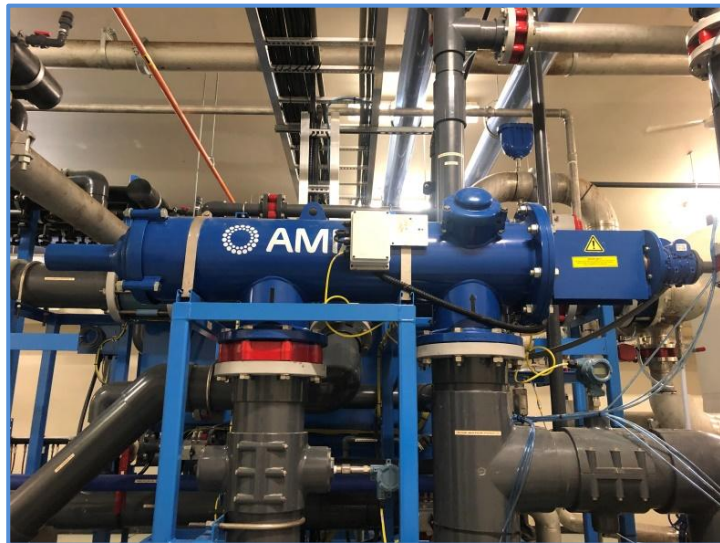
Figure 3. Self-cleaning Strainer
