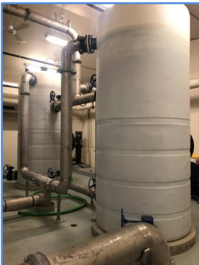
Figure 2. Balancing Tanks
