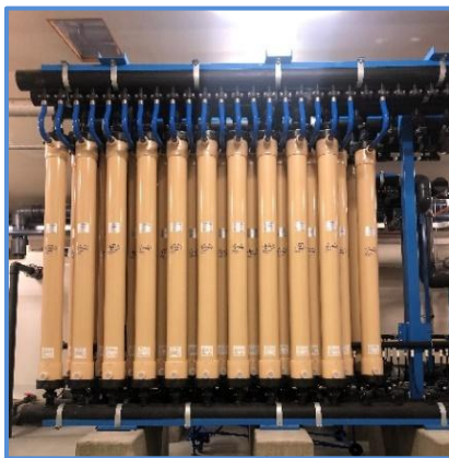
Figure 4. Microfiltration Modules
