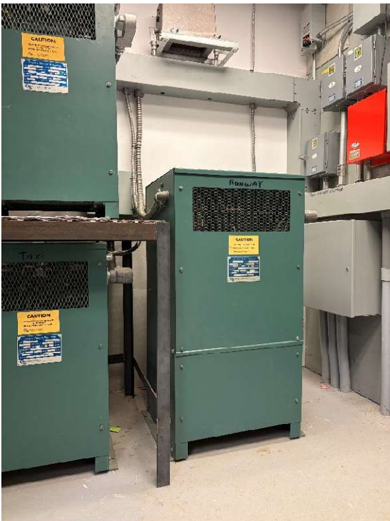
Constant current regulator for runway lights.
